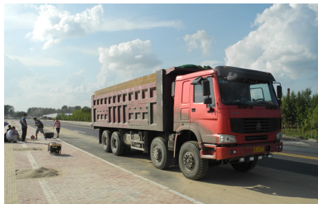
图 14 B 场地现场测试试验图 Fig.14 Field test on site B
